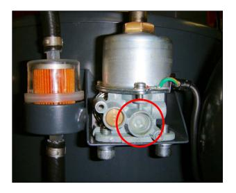
**8.** If the filter is dirty remove it with a small screwdriver and clean with hot soapy water and replace, making sure it is dried completely first.
