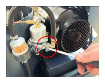
**19.** You will then need to run the machine up to bleed the pump and obtain pressure on the gauge between 100-110 psi to ensure the correct burn.
