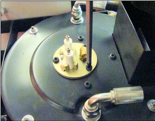
**16.** Replace burner head back into boiler and fix with 3 x M6 screws.
