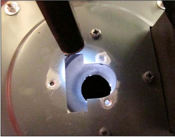
**15.** Whilst burner head is removed check the inner lid and cone with a torch for damage. If damage has occurred to inner lid and cone, stainless steel pan or inner boiler these items will need replacing as they effect the burning of the boiler. (See How to replace a boiler)
