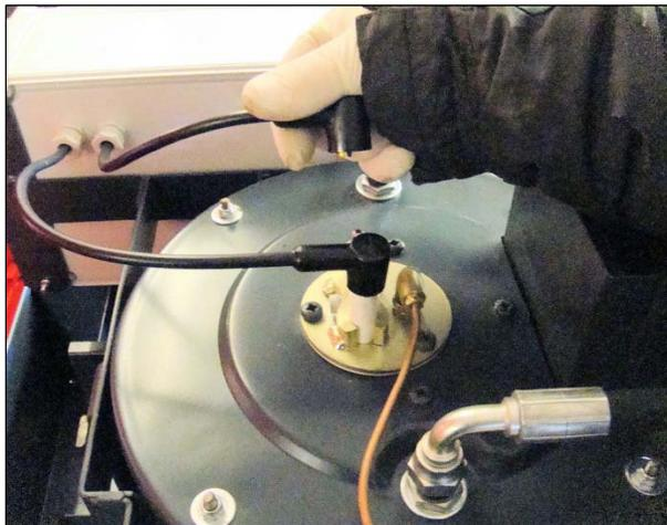
**10.** Moving to the top of the boiler. Disconnect HT leads from electrodes and move to one side.
